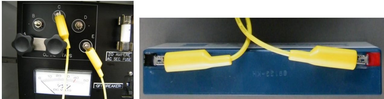
Figure 18 uGI1 Power Connections (AC voltage from rectifier taps or DC voltage connections)
